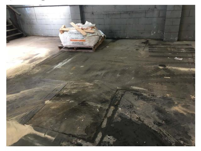
**Photograph 1:** Concrete patched area found at the rear portion of the existing service centre (20 April 2018).
